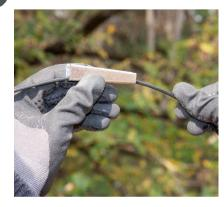
Position the shim onto the cable in the clamp's body, with the gripping bumps facing the cable.
